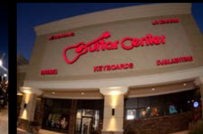
Guitar Center Complete Remodel 2026
